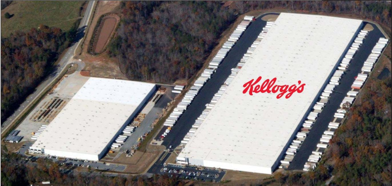
The Kelloggs Distribution Center is a new 903,000 SF food grade distribution plant located in Atlanta, Georgia. Construction of this project included load bearing concrete tilt-up panels with interior structural steel columns, a steel frame roof structure, heavy duty reinforced floor slabs, and ESFR sprinkler systems. The facility also includes 18,000 SF of office space and high pile storage in racks. RACO was awarded the contract as Design-Build Prime Contractor.
